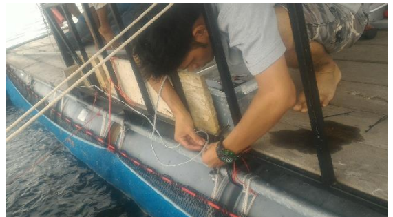
Figure 8 The installation of water quality sensors
