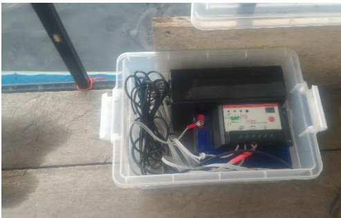
Figure 6 The installation of the system
