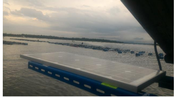
Figure 7 Solar cell installation
